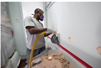
A contractor blows cellulose insulation into the walls of a home.
